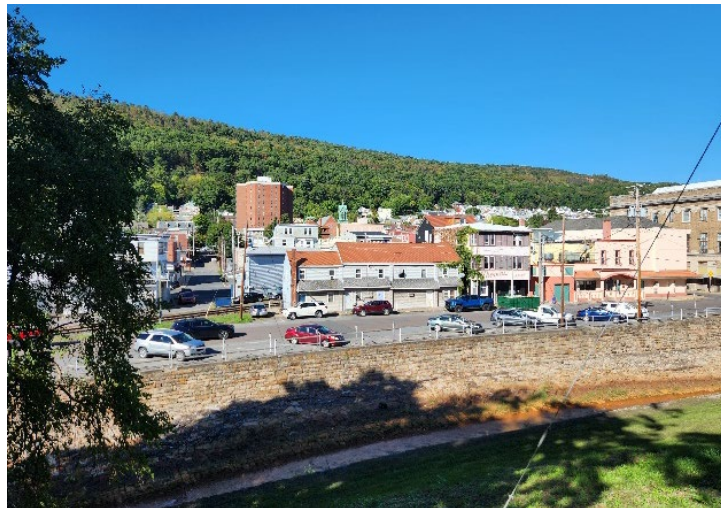
FIGURE 7 RETAINING WALL BELOW WATER STREET ADJACENT TO SHAMOKIN CREEK
