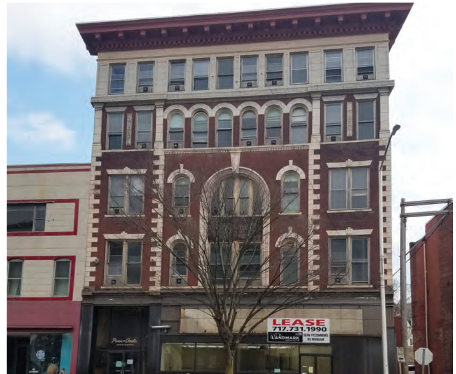
Former Rennas Hotel Building
